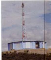
The Pierre Auger Observatory combines techniques used in earlier experiments to study cosmic-ray air showers at the highest energies. Water tanks, such as the one on the right, detect Cherenkov radiation produced by charged particles, while on dark nights optical detectors housed in larger buildings (left) record the faint light emitted as the showers cause fluorescence of atmospheric nitrogen. (Photos: Pierre Auger Laboratory.)
